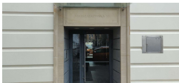
Figure 5: Entrance to the building from the courtyard.
